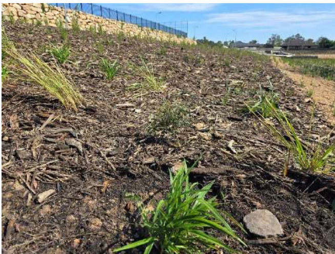
Photo set 8: Rehabilitation and erosion and sediment control measures through drainage areas on site.
