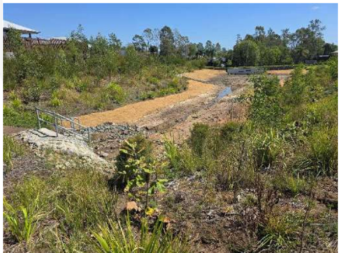
Photo set 8: Rehabilitation and erosion and sediment control measures through drainage areas on site.
